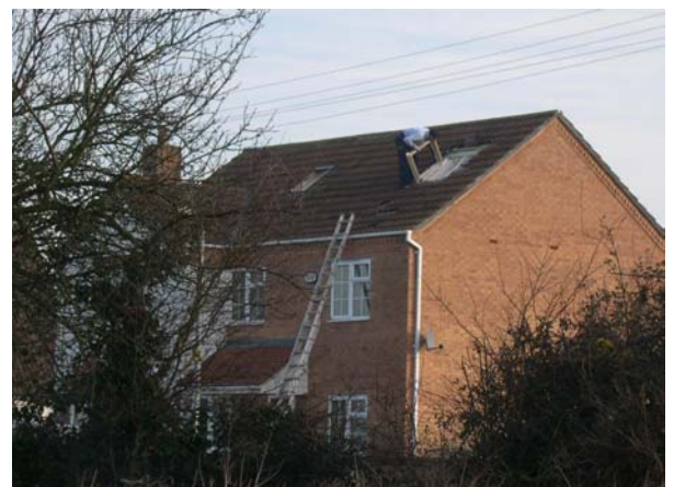
Installing a window in a roof without edge protection
