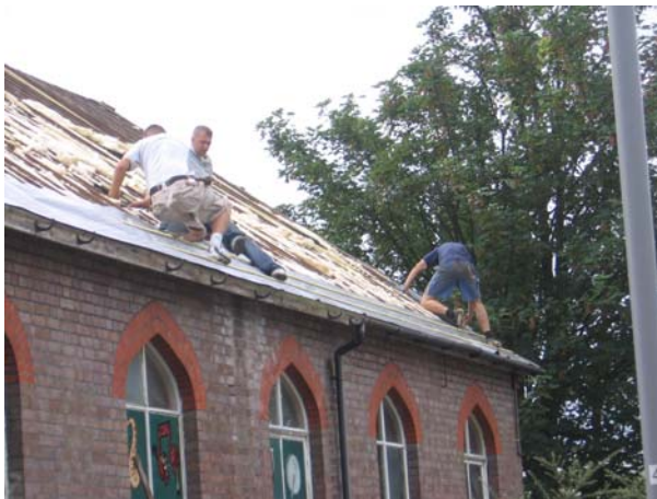
Constructing a dormer with insufficient scaffolding
