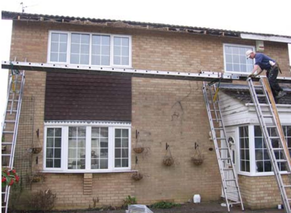
Reroofing a sloping roof without scaffolding
