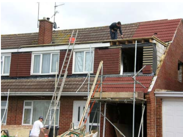
Constructing a dormer with insufficient scaffolding
