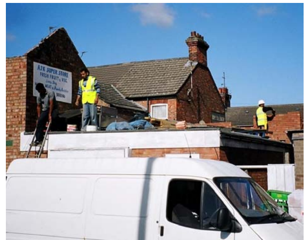
Installing a window in a roof without edge protection
